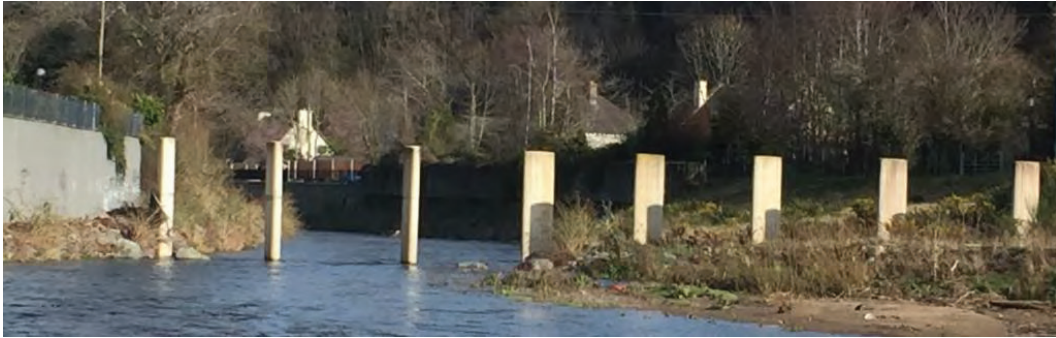
Figure 4.19: Example of Debris Trap
