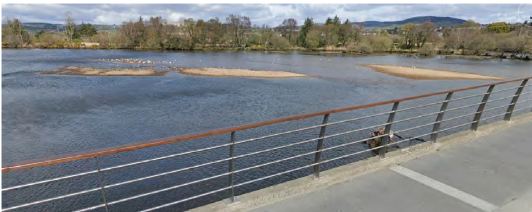
Figure 4.13: Sandbanks Upstream of Arklow Bridge
