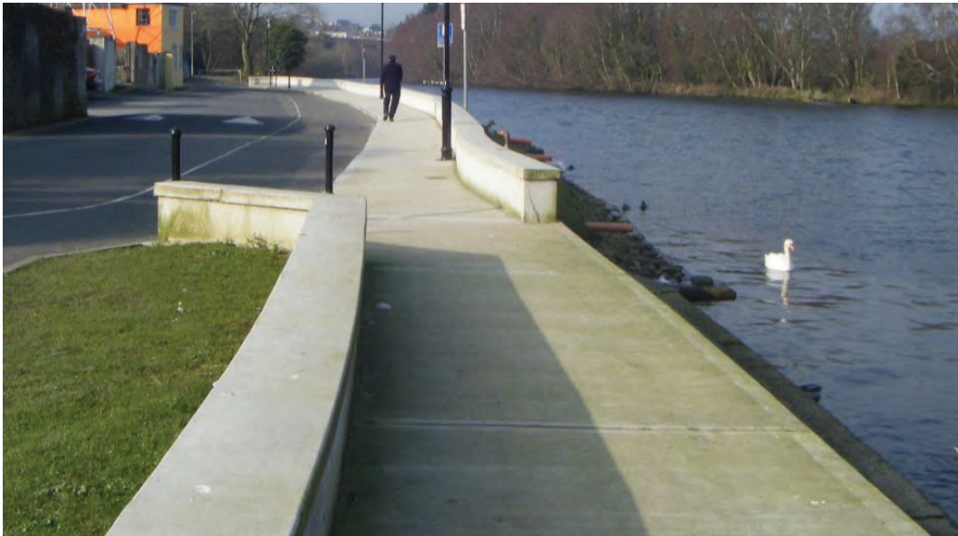
Figure 4.22: Existing River Walk Footpath and Wall
