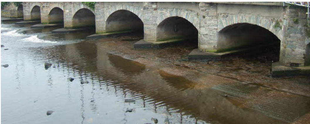
Figure 4.9: Existing Scour Protection Slab
