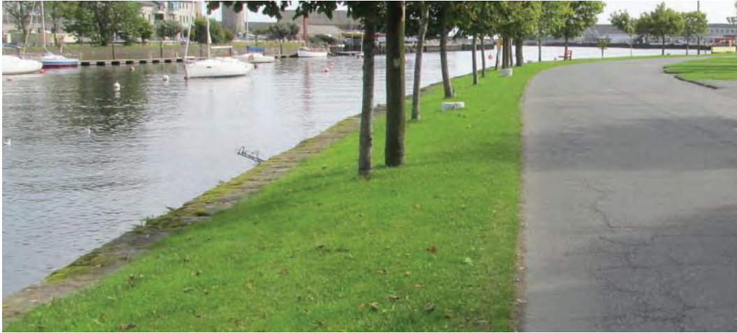
Figure 4.25: Existing Open Quay on South Quay, downstream of Arklow Bridge
