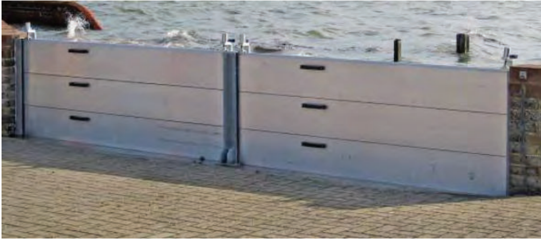
Figure 4.30: Example of Demountable Flood Barrier
