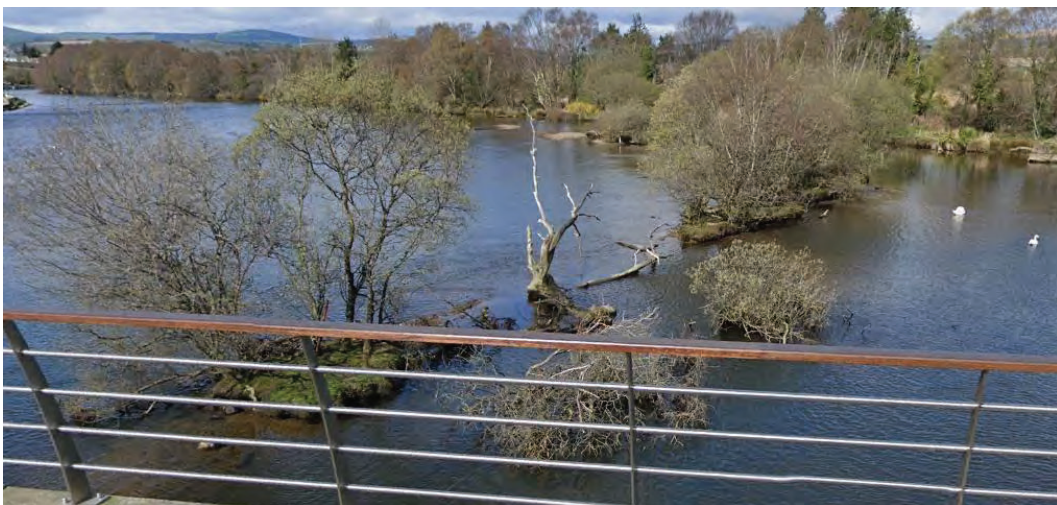
Figure 4.15: Vegetated Islands Upstream of Arklow Bridge
